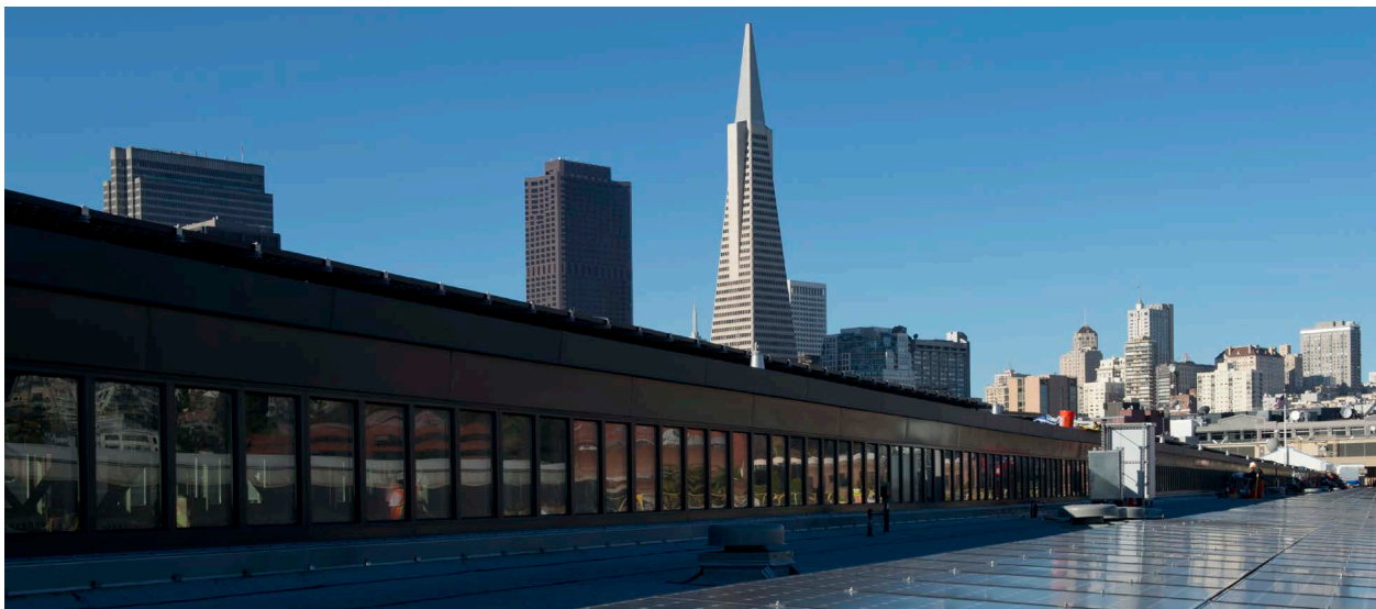
Photo: San Francisco Exploratorium Renovation
